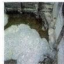
Foaming, dirt and sludge
