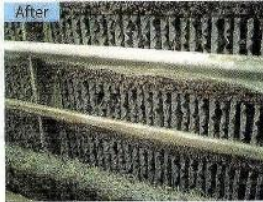
Algae completely removed from tower infill after 1 month installation of Sora Treatment System
