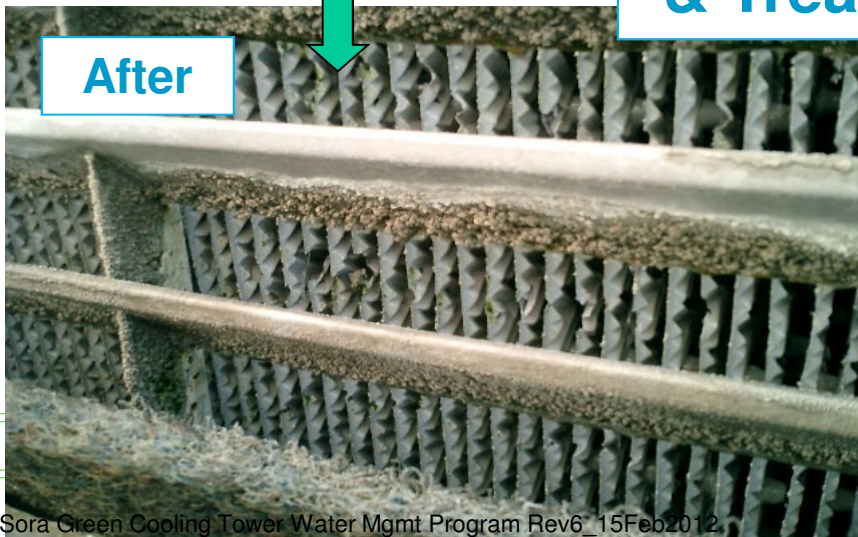
Cooling tower infill fouling & algae growth (after 1 month)
