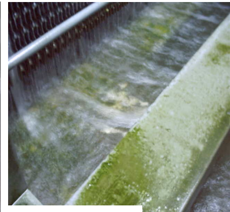
Foam, dirt, sludge at cooling tower basin due to interaction of chemical cocktails
