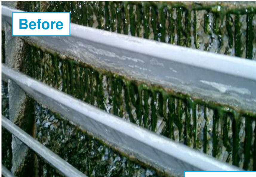
Cooling tower infill fouling & algae growth (after 1 month)
