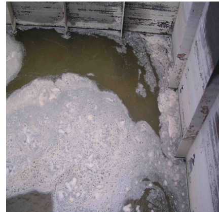
Foam, dirt, sludge at cooling tower basin due to interaction of chemical cocktails
