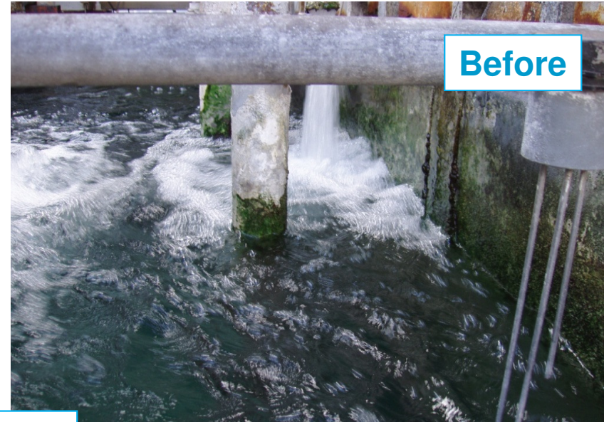
Cooling tower basin slime & algae growth (after 1 month)
